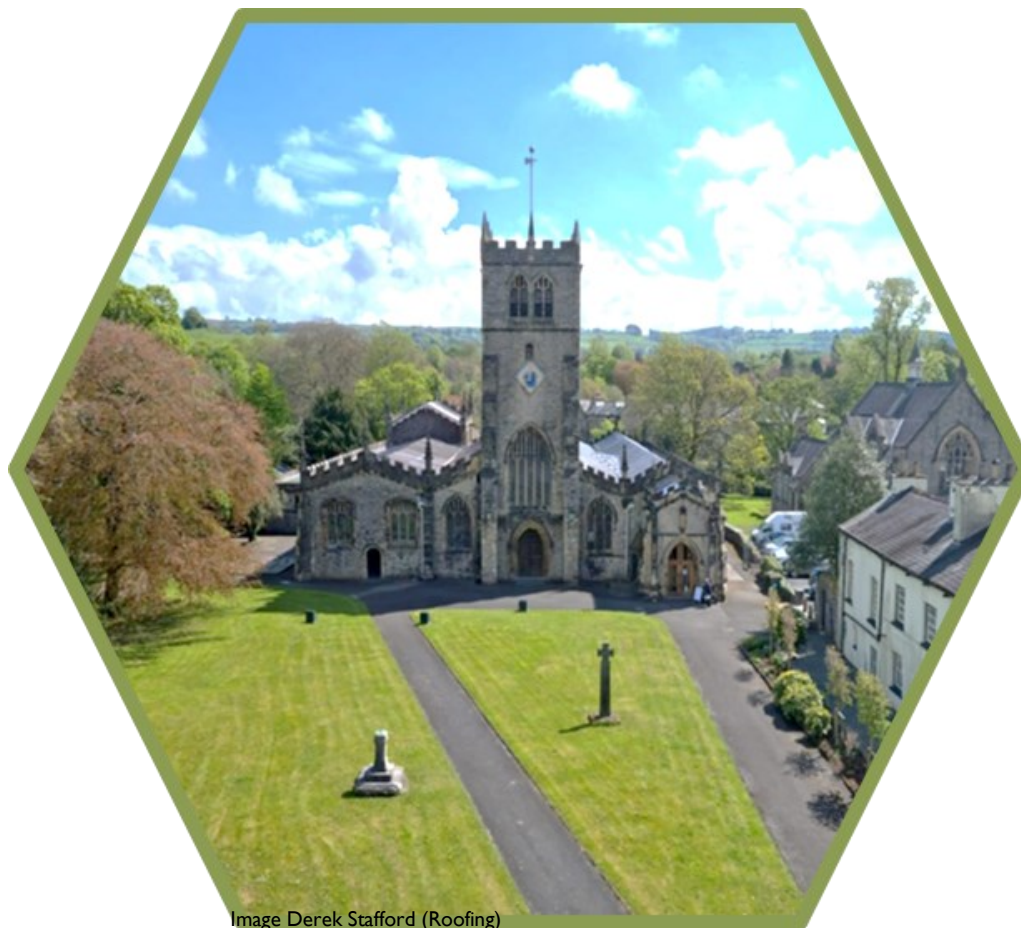
Image Derek Stafford (Roofing)
