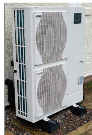
'Green': New features include solar panels and, right, and an air source heat pump
