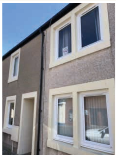
External painting and new windows
