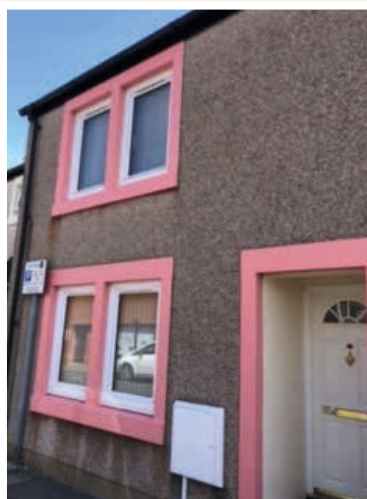
External painting and new windows
